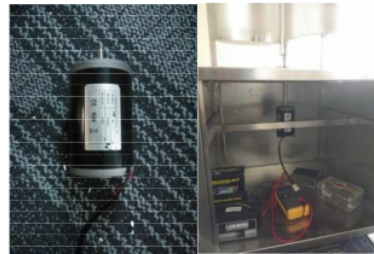
Fig. III.7. 1 st Generator Implementation
